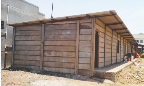
Precast Labor Quarter
