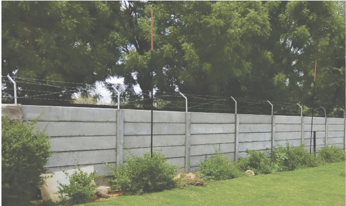
Precast Pre-stressed Wall With Barbed Wire Fence
