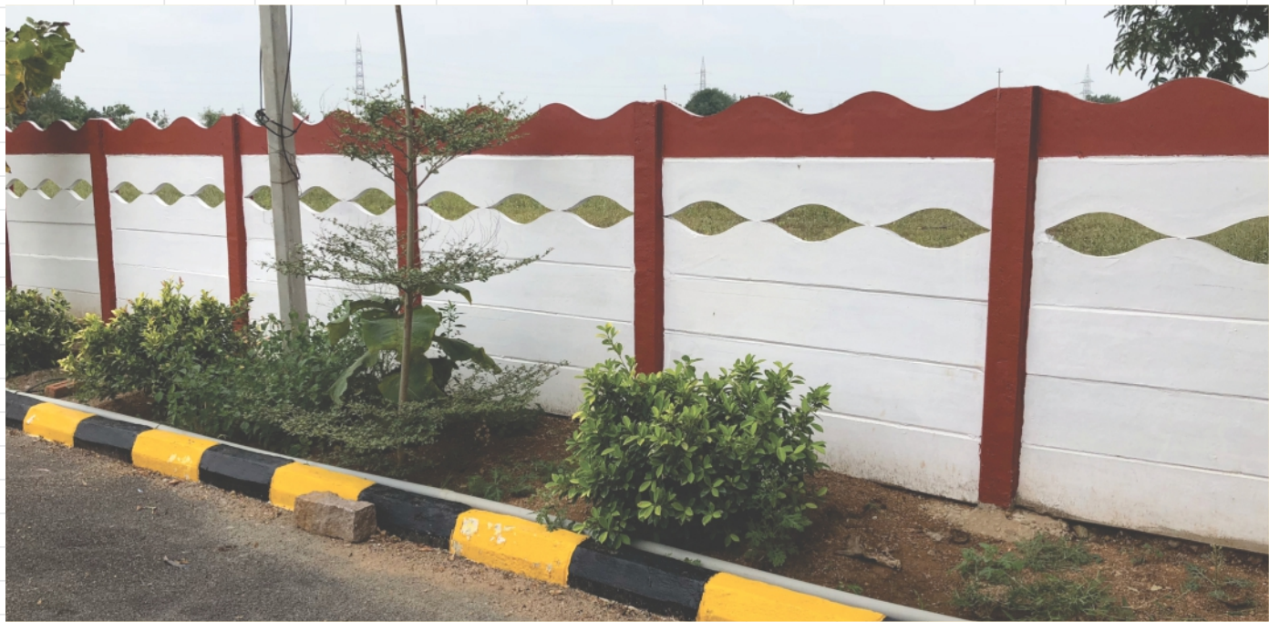
FARMHOUSE COMPOUND WALL
